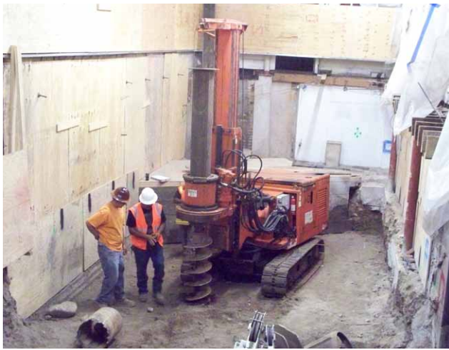
Figure 5 Pile drilling in a confined space inside the Hammel Building. Photo: City of Los Angeles
