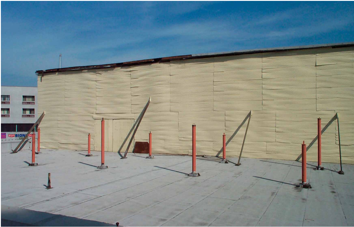
Figure 1 One of a series of protective coverings erected over the mural since 1982. The steel columns in the foreground were intended to support a future mural shelter. Photo: Brooks + Scarpa
