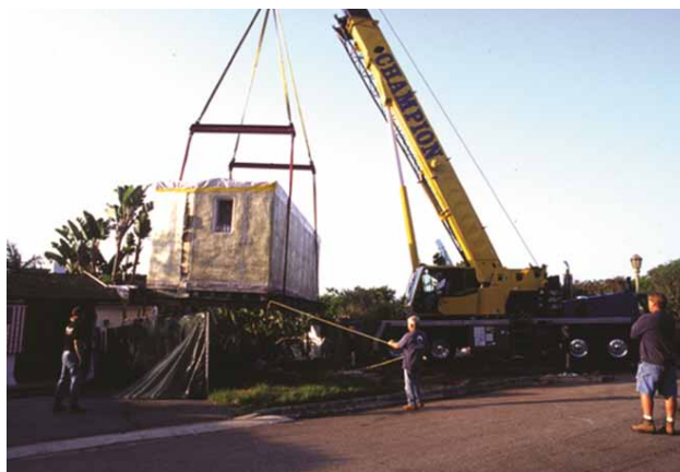
Figure 5 Ted Hollinger of Master House Movers and his crane operators, on site in Pacific Palisades, lifting the twenty-five-ton mural-building onto a lowboy tractor-trailer headed for Santa Barbara. Photo: Siqueiros Mural Project Team, Courtesy Santa Barbara Museum of Art
